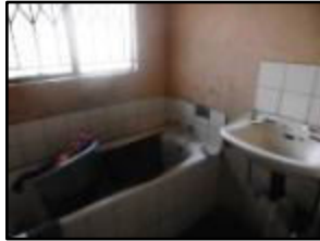
Bathroom with bath and basin.
